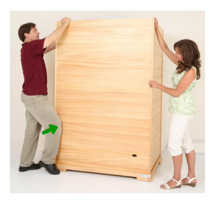
Connect the Back Wall to the two Side Walls Position the back wall by wedging it into the channel in the floor base.
