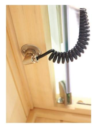
Connect circular connector for the door heater.
