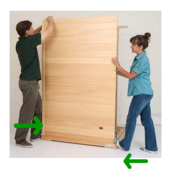
It is helpful if a second person applies pressure against the opposite edge of the back wall. This will helps ensure that the two walls remain in contact and the fasteners will connect.
