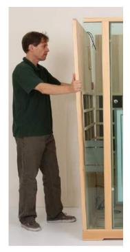
Insert the Left Side Wall into the channel of floor base while aligning the slot in Side Wall with edge of Front Wall glass panel.
