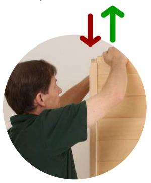
Slide the Back Wall up approx. 3/4" while holding the Side Wall down with your opposite hand. The 2 sets of fasteners for the walls will connect when the back wall is raised sufficiently. When you feel the fasteners connect, slide the Back Wall back down.
