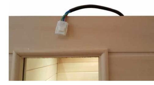
Ensure that the electrical wire protruding from the top of the front wall is flipped to the outside of the sauna.
