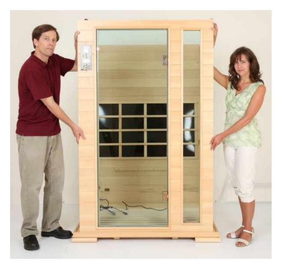
Position the cut-out in the bottom of the front wall over the wires protruding from the floor base
