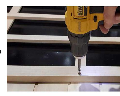
Install screws to firmly attach heater guard to the wall
